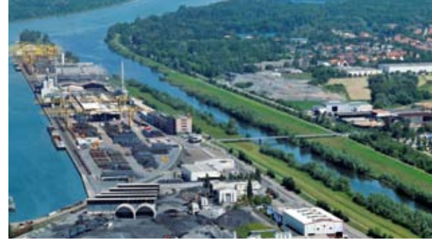
Kehl/Rhine, Germany: aerial view on one of the world's most successful EAF steel plants.
