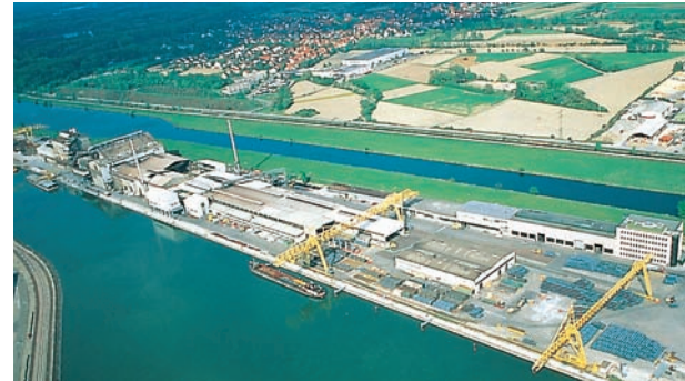
Kehl/Rhine, Germany: aerial view on one of the world's most successful EAF steel plants.
